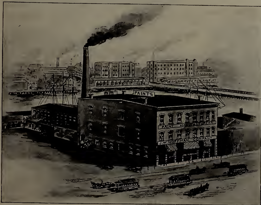
PAINT WORKS OF THE J. W. HOFFMAN COMPANY, 436 to 440 Atlantic Avenue.
